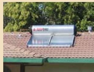
**Solar Water Heater.** These systems do not convert solar energy into electricity, but rather use the sun's rays to heat water.
