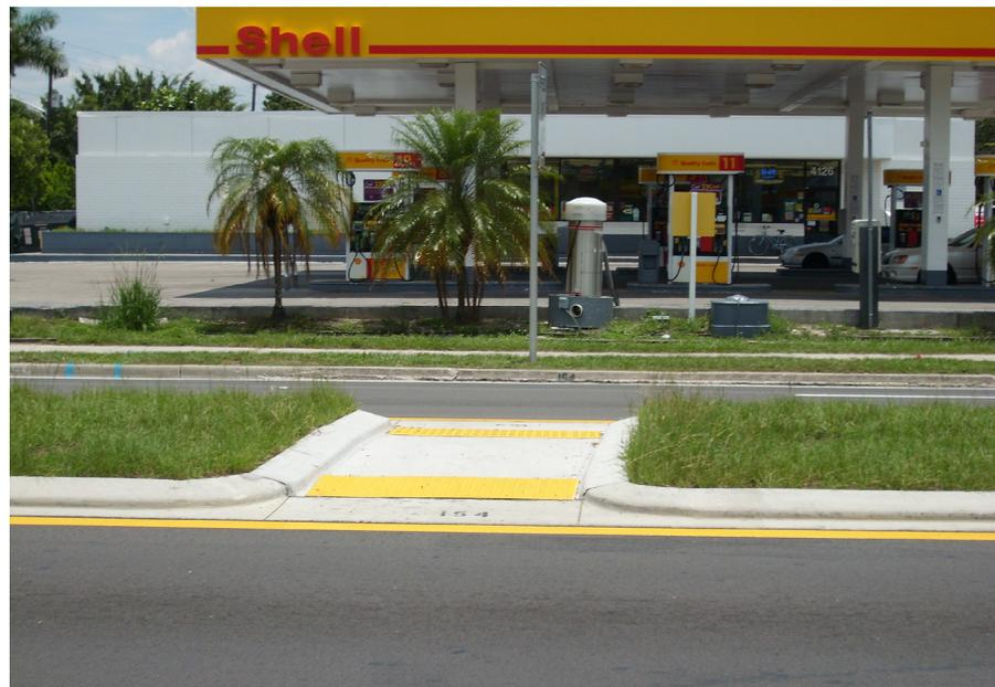
Figure 5.7: Median pedestrian crossing; opposite curb does not have a ramp for wheelchair access.
