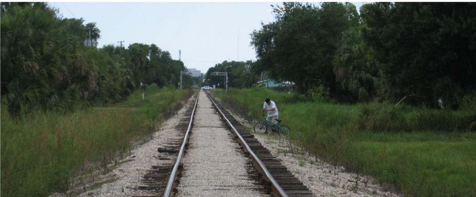
Figure 1.7: Poorly maintained rail lines and right-of-way.
