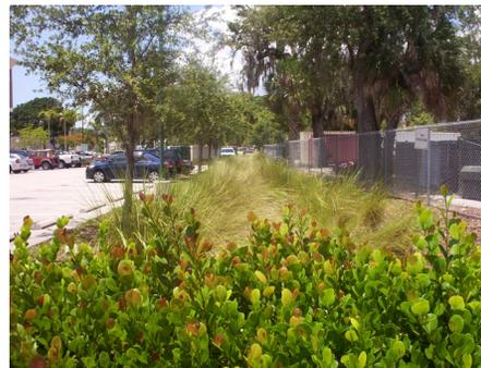
Figure 6.18: Drainage swale planted with natives
