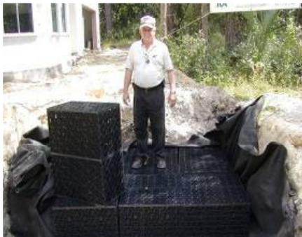
Figure 6.17: Exfiltration tank
