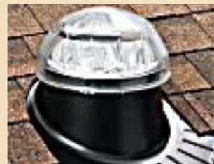
**Solar Tubes** channel sunlight into window-less rooms, to reduce the need for electric lighting.
