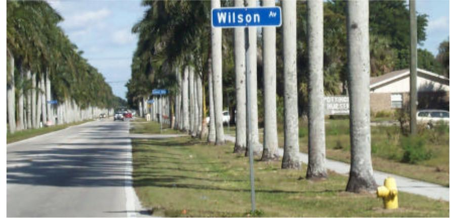
McGregor Boulevard, Fort Myers, FL. An example of an open drainage swale that has been replaced with a pipe and shallow swale. The layout of the swale, street tree line, and sidewalk is similar to what has been proposed for the avenues of Naples Park.
